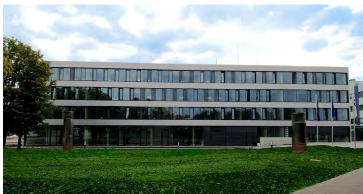
Figure 10: View of the new EOC at DLR in Oberpfaffenhofen
