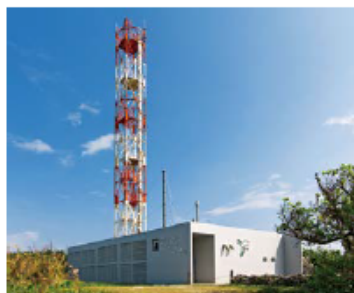
Monitoring station, Hateruma
