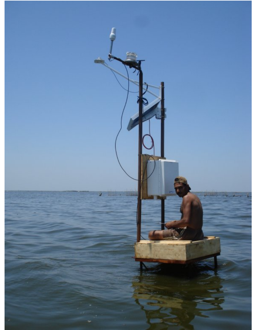
Installation of one of the in-situ stations in August 2009.
