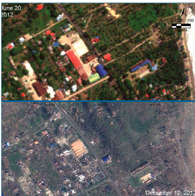
Figure 1: Example of a satellite EO-based product using optical imagery comparing an area before (GeoEye satellite) and after (SPOT satellite) the landfall of Typhoon Bopha in the Philippines in December 2012. It is worth noting the damage to buildings and tree plantations.
