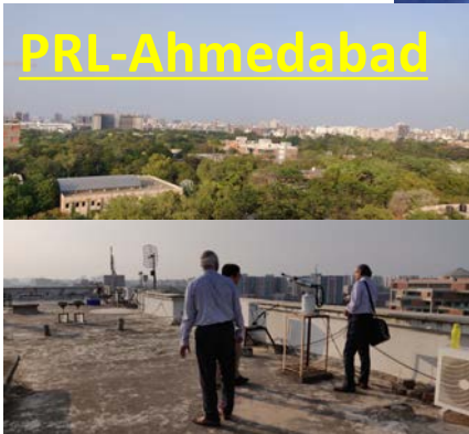
Roof of the building at PRL
