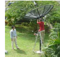
CATHALAC/SERVIR Antenna Installation
