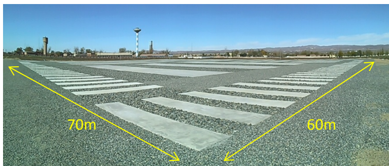
Finished construction by the end of September, 2014
