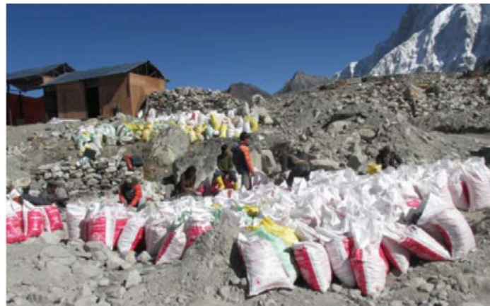
Breaking of stone for aggregate collection
