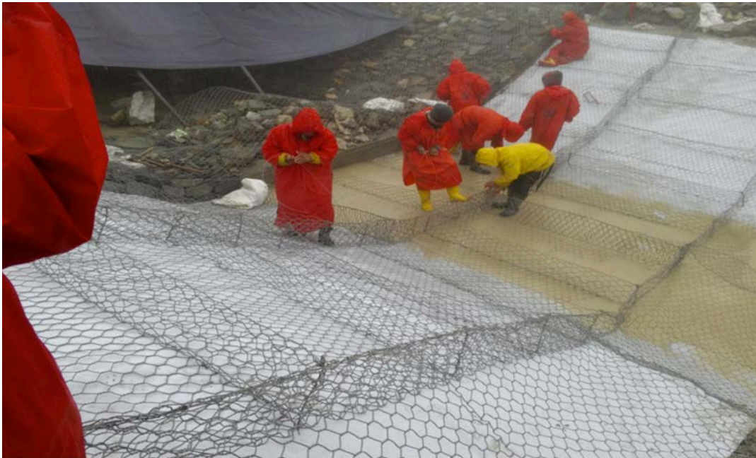
Reno mattress work in d/s of gate.
