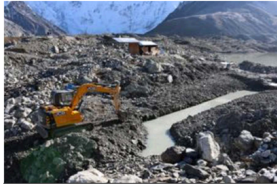
Excavated main channel
