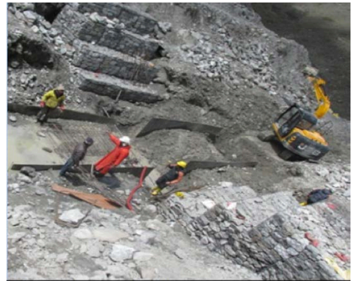
Excavation work of cutoff.
