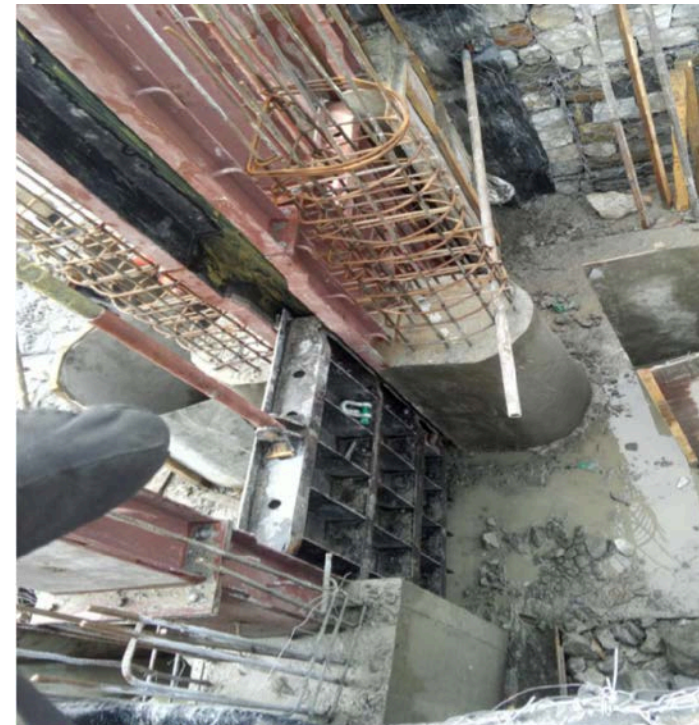
M25 Concrete in column section,
