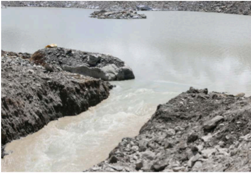
Water flowing through diversion channel.
