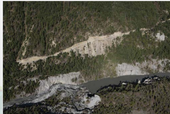
Figure 15. Aerial image of the Pisang 2 earth slide along the Marsyangdi River upstream from Pisang village. As of May 30, 2015, this landslide constricted the river with a 350-m-long slackwater lake upstream of the landslide deposit. Maximum width of impoundment in image is approximately 50 m.
