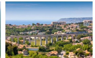
6e SCO France meeting: the rails are laid Read more
