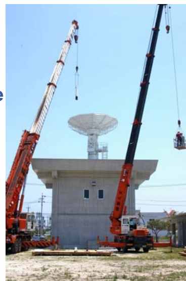
First installation: Japan
