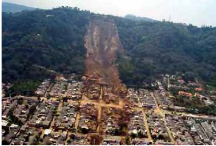
FIGURE 14: LANDSLIDE COLONIA LAS COLINAS (EL SALVADOR) PICTURE CREDITS: USGS (ED HARP)
