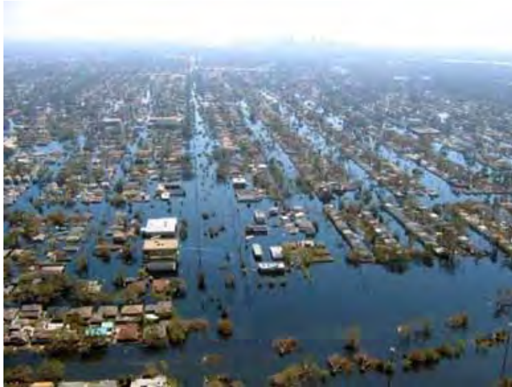
FIGURE 4: FLOODING IN NEW ORLEANS AFTER HURRICANE KATRINA, 2005 © NOAA
