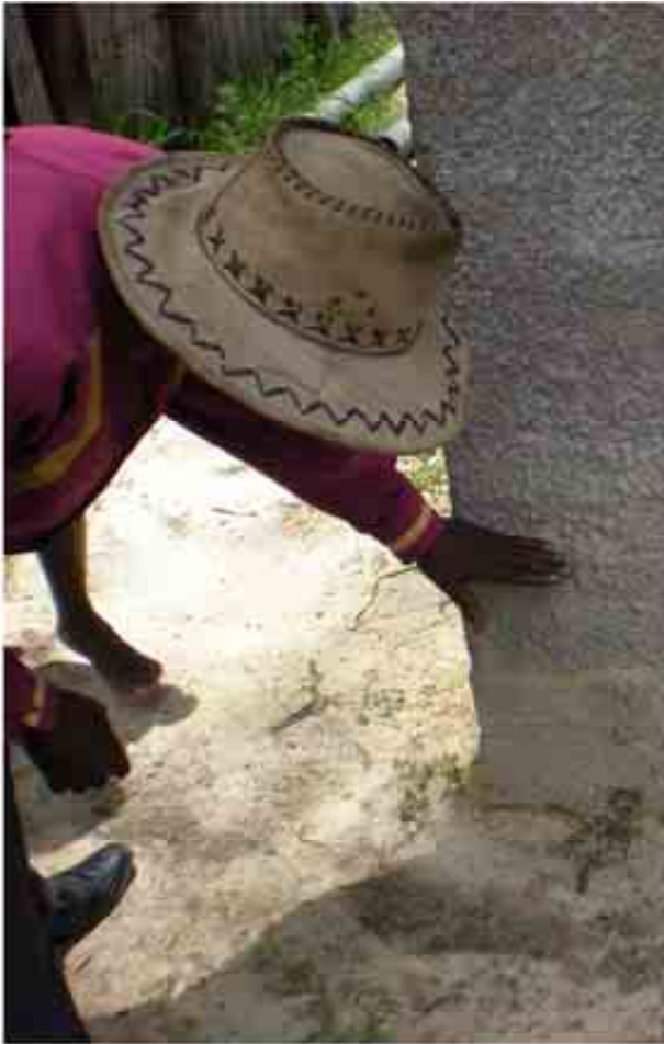
Villager shows flood damage and impact during team site assessment
